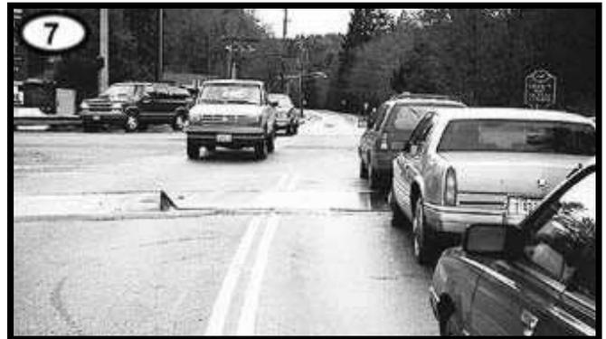
Steel construction plates can be as slippery as ice when they are wet. And their sides often form edge traps as well. Sometimes, even worse, they don't always cover the hole. Don't drop in for a visit.
